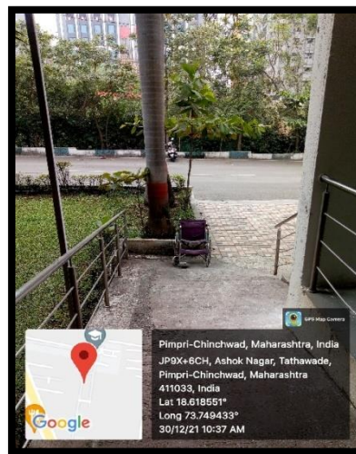
Ramp and Railing
